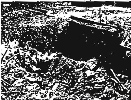
Test pit located between 8 and 9 shows void.
