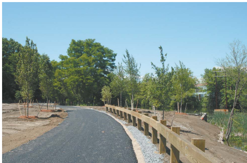
Another view of the park under construction.
