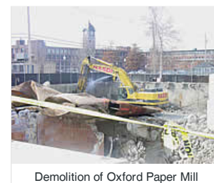
Demolition of Oxford Paper Mill
