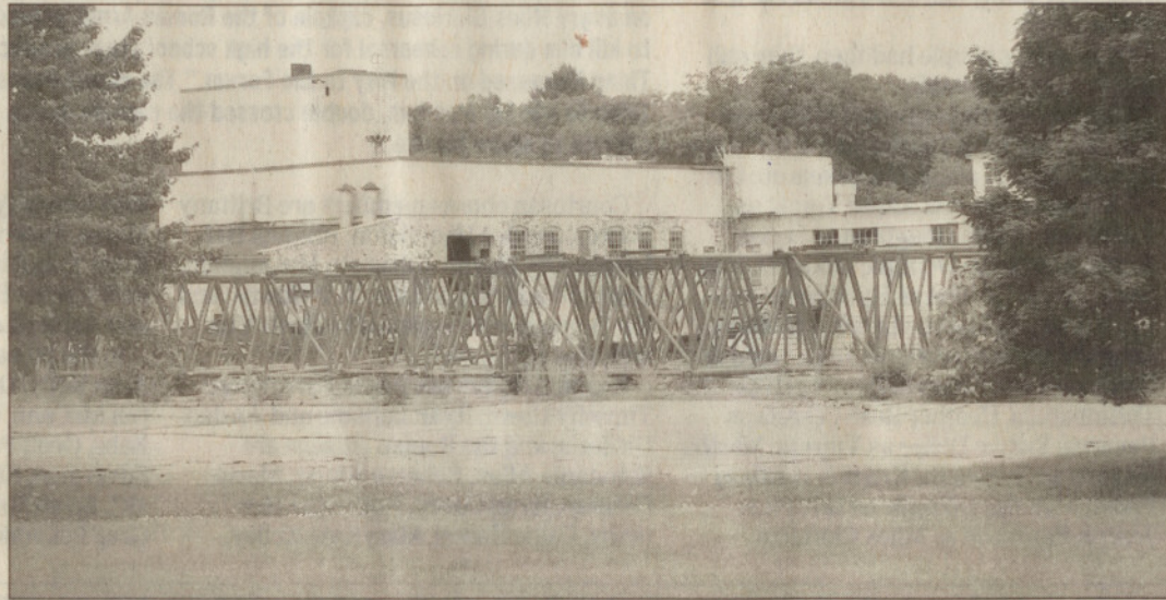
The Reichhold Chemical site in Ballardvale was being cleaned up in spring 2004.
