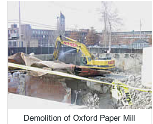
Demolition of Oxford Paper Mill
