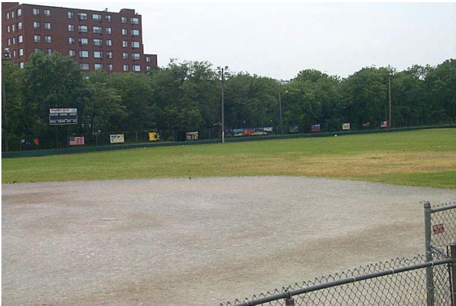
Existing Playfield: Poor drainage after flood event
