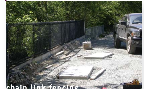
chain link fencing
