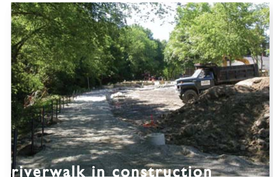
riverwalk in construction
